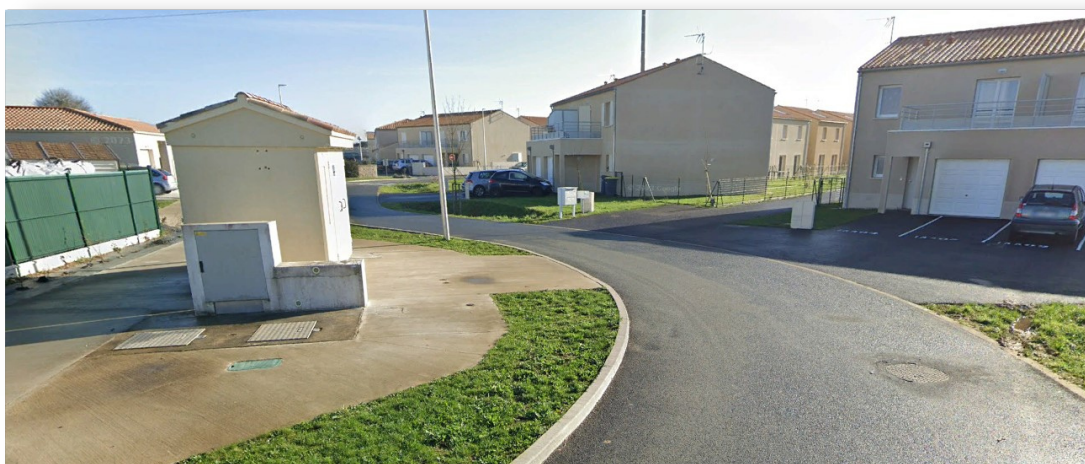
Source : Station de relevage Echillais
